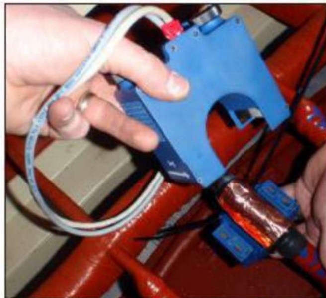
Figure 7: Assembling a Current Transducer Head on a winding link of an Electrical Generator Stator. Reprinted by permission from the USBR.
