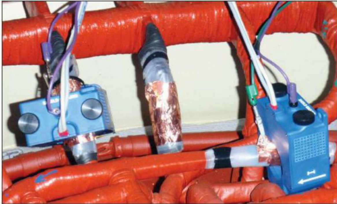
Figure 6: Application on Electrical Generator Stator. The two Current Transducer Heads are shown installed on the winding links. Reprinted by permission of the US Department of the Interior, Bureau of Reclamation (USBR)
